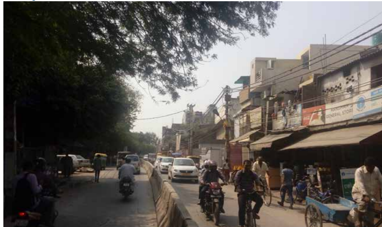
General Existing Section of IGNOU Road
